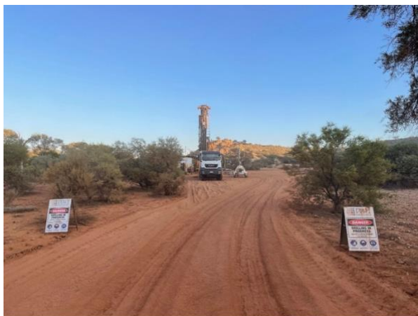
Figure 31 – Drilling equipment on site at drillhole
