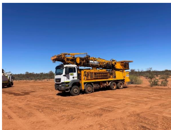
Figure 29 – Arrival of drilling equipment
