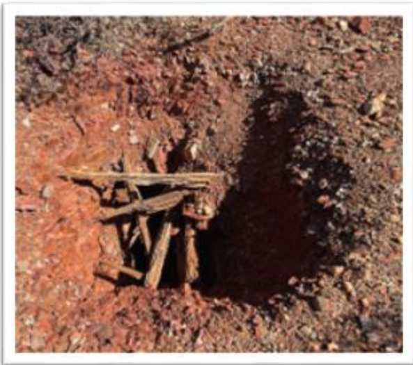
Figure 17 - Historic Eastern shaft observed at the Gorge Mine Prospect.
