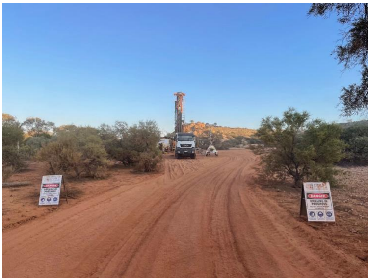
Figure 31 – Drilling equipment on site at drill hole JUD002
