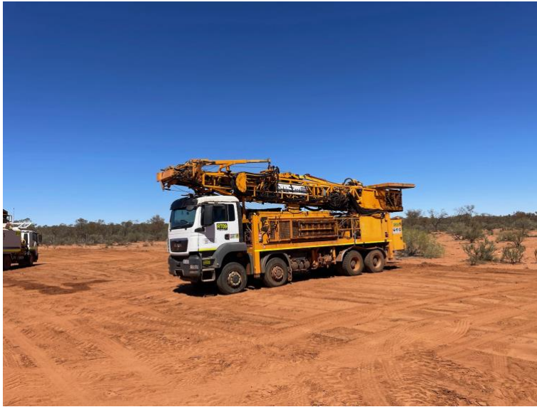
Figure 29 – Arrival of Drilling Equipment
