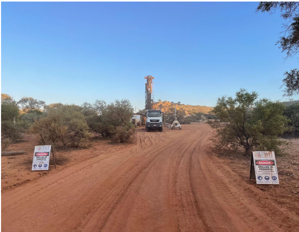
Figure 1 – Drilling equipment on site at drill hole JUD002
