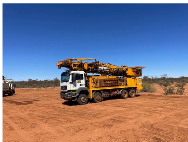
Figure 6 – Arrival of drilling equipment
