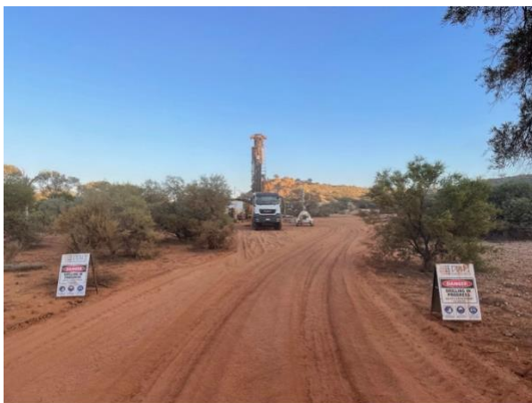
Figure 8 – Drilling equipment on site at drill hole
